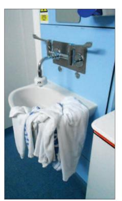
A handwash basin used inappropriately for storage of used towels. Note the point-of-use filter fitted to prevent the release of Pseudomonas aeruginosa due to repeated colonisation of the outlet.
